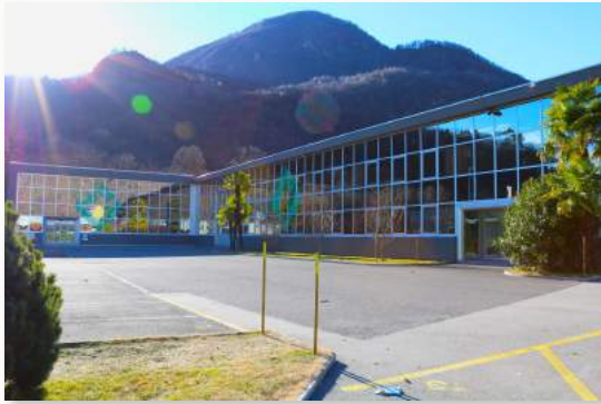
Newly built infrastructure with a state-of-the-art construction design and high security.
