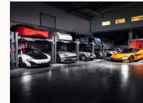
Secure double-height spaces accessible h.24
